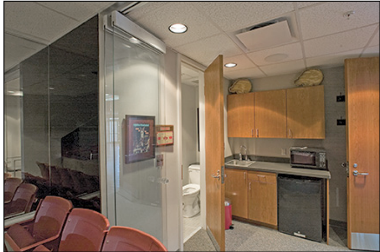
INSIDE ONE OF THE 12 LUXURY SUITES AT BUD WALTON ARENA: INSTEAD OF CONVENTIONAL PLUMBING, THE WET BAR AND PRIVATE RESTROOM USE SANIFLO ABOVE-FLOOR PLUMBING TECHNOLOGY
